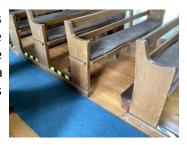
3.8 Pews are very simple benches which have been modified following the modification of the floors. This has created a trip hazard when entering the pews. This is currently marked with hazard tape, but it would be a desirable improvement to consider other options for this.
