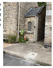
4.27 Although pretty, the vegetation along the front wall is likely to hold moisture against the building. It should be removed to help resolve the issues of damp within the church.
