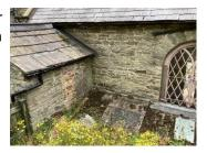
4.17 Both the Vestry and northern window would benefit from redecoration, and the northem window from repair. When repairs are undertaken to the northern window, attention is required to improve the flashing detail to the area. It is currently flashed with a mixture of flash band and lead flash band, which while flexible has a very short life span. Consideration might be given to reinstating the full northem window to resolve this detail more fully.
