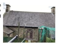
4.1 There are several slipped slates on the under course which are now sitting in the gutter on the north side. These should be removed from the gutter and refixed.
