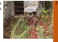
4.21 The stonework to the eastern elevation is generally in fair condition. Pointing is reasonably tight and while there is a small amount of hard mortar pointing, the stone is holding up well at present.
