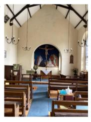
3.1 The roof consists of slender scissor trusses with no bottom cord, intermediate purlins, and plastered between. There is a little discolouration at each of the gable ends. It is assumed that this is the result of moisture coming from the walls where there have been problems in the past. Once the walls have dried the area can be redecorated with a breathable paint. There are no other signs of damp within the roof structure.
